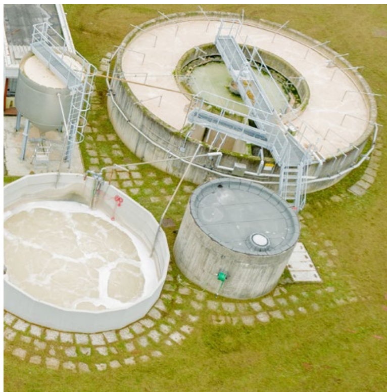
Wastewater treatment plant Origgio Site
